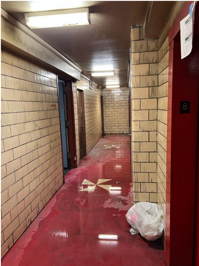
The three photographs above depict hallway flooding that resulted from overflows of sinks or broken pipes from inside apartments. The first photograph in this series is the top of an elevator car that was soaked by water. Once water enters the shaft and onto elevator equipment, the elevators are generally out of service for several hours while the water is removed, and equipment dried.
