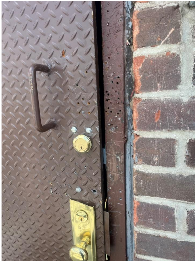
The photograph above shows a EMR exterior door that was damaged in the process of someone forcibly opening the door to gain entry.
