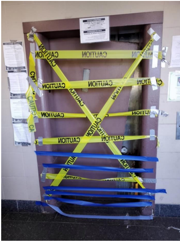
These photographs above depict a recently vandalized elevator door that was damaged to such an extent that the door became partially detached from the elevator car. When discovered, the elevator was closed off and out of service for several days until the door could be properly reattached.
