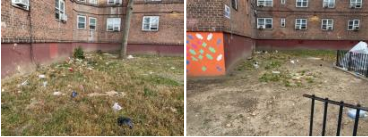
Photographs of trash that appears to have been thrown from apartment windows. The field examiners have noticed dangerous objects, such as glass bottles, that appear to have been thrown from windows onto the ground below causing safety issues for NYCHA residents and staff.
