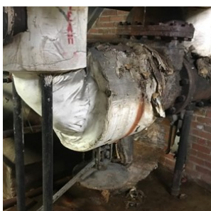
Corroded steam trap; the deaerator for this steam system needed to be replaced so the gases in the water could be removed
