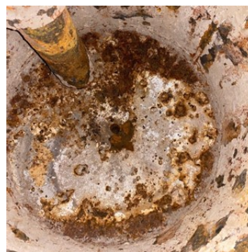
Inside of a steam boiler blowdown tank after decades of use
