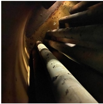
Inside of a steam boiler used for humidification. The brown colouring is a natural magnetite layer
