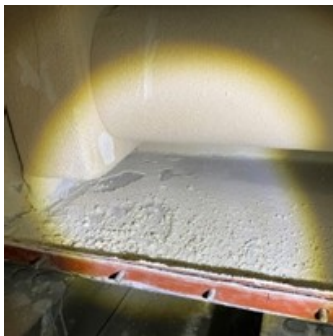
Scale build up over time inside of a humidification unit
