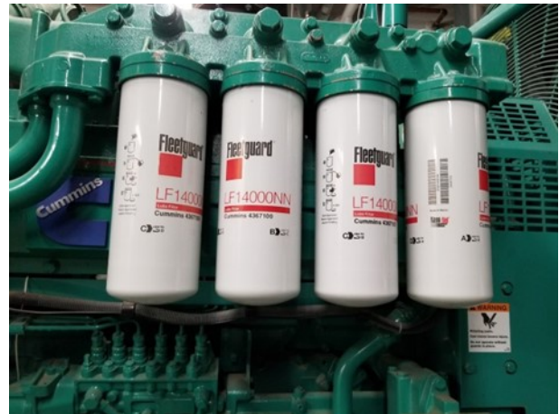
Best practices dictate that lube filters should have the date of change written on them with a Sharpie
