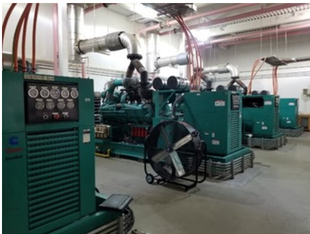
Clean and well maintained Cummins KTTA50-G2 1500kW 4160v
