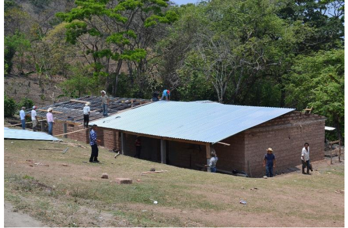
Men from the village of La Laguna building three new classrooms.
