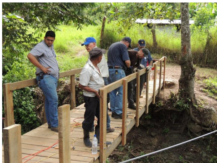
Rotarians building a footbridge in the village of Nuevo San Isidro, so that students don't have to wade through a waist-deep river to get to school during the rainy season.
