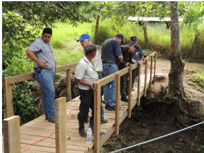
Rotarians building a footbridge in the village of Nuevo San Isidro, so that students don't have to wade through a waist-deep river to get to school during the rainy season.
