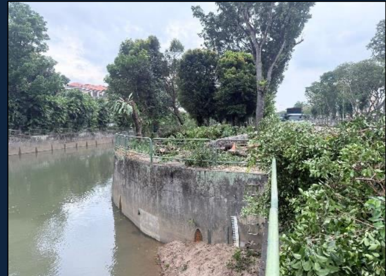
Excavation Process to expose the pipe
