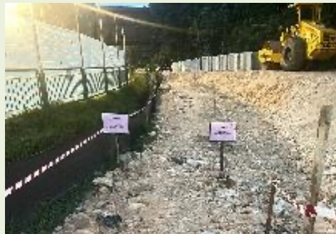
Water pipe alignment tagged and demarcated on site
