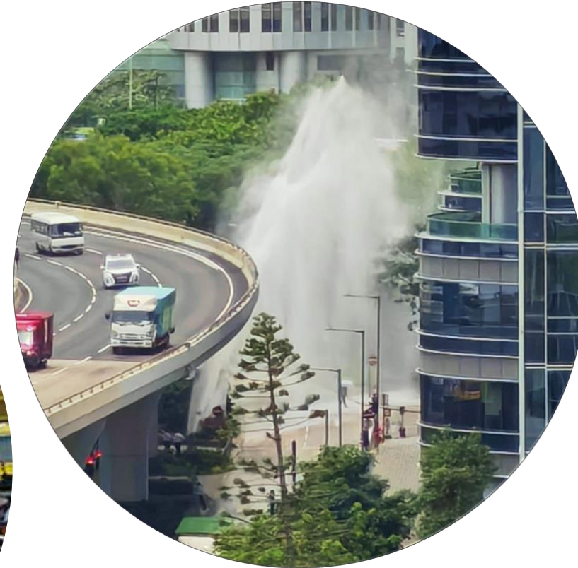
Aging problem of water pipes
