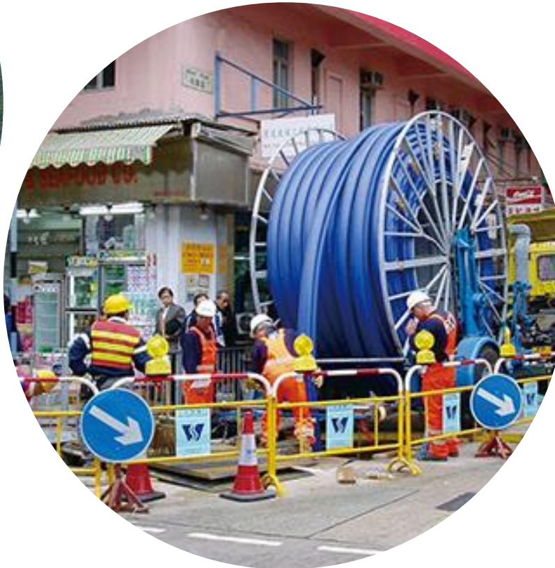
Congested urban setting and underground utilities services
