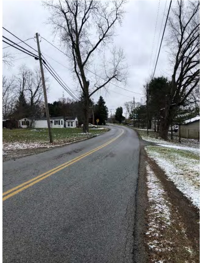
Faulkner Road Looking East
