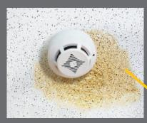
Stains on interior ceilings and walls or mold and mildew growth. Possible causes: Inadequate or faulty shingle underlayment allowing leakage, or inadequate ventilation.
