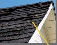
Missing, cracked, or curling shingles. Possible cause: Shingles have reached the end of their useful life.
