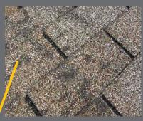
Dark, "dirty-looking" areas on your roof. Possible cause: Loss of granules due to age of shingles.
