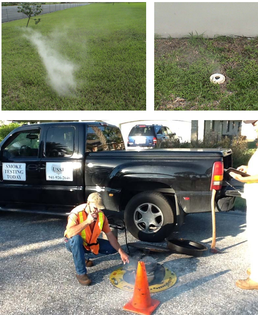
Figure 8. Smoke test results.
