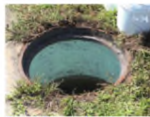
Frame & Chimney – Prime Coat
