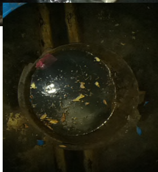
Figure 3a Grease in the manhole 3b. Improper disposal of material 3c Wipes 3d Old manhole dish
