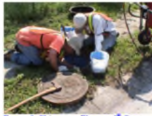
Frame & Chimney – Elastaseal® Coat
