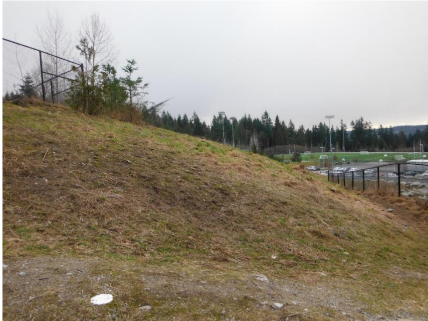
Photograph 1: Cut banks between western disposal field and SD 43 infrastructure. Disposal field is at grade with fencing in top left corner. Cut banks are tiered (fencing to the right is top of second tier, see next photograph)
