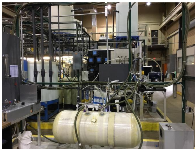
Figure 1: Mock aircraft water system constructed at EPA's Test and Evaluation Facility in Cincinnati, Ohio.
