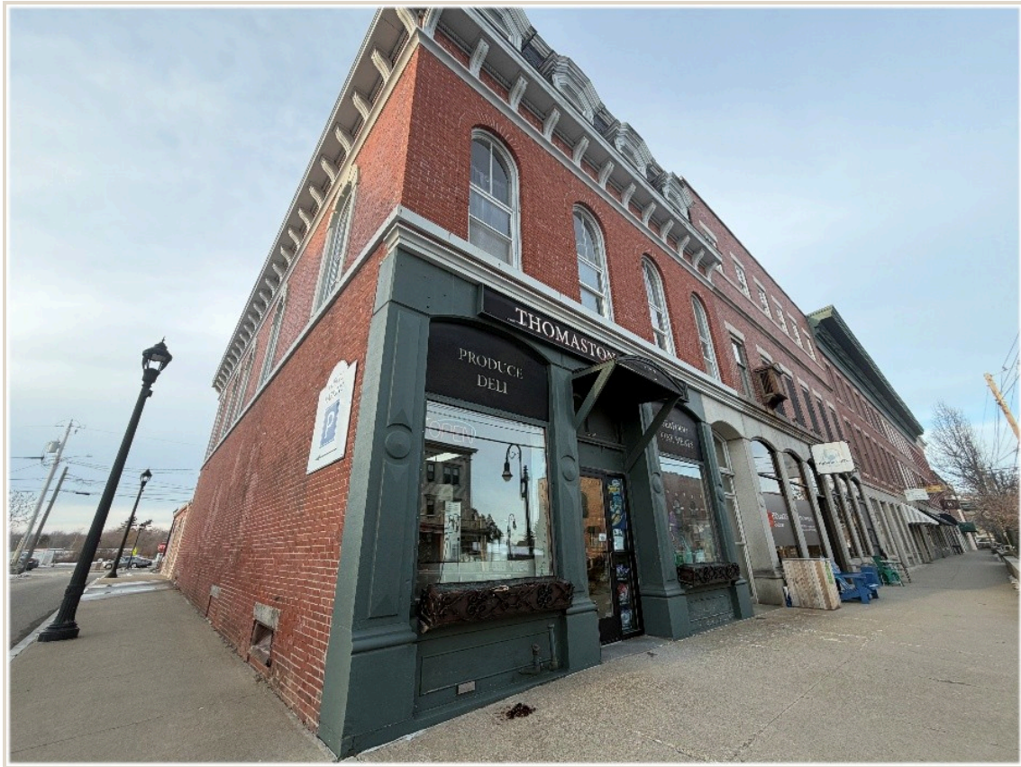
Thomaston Grocery — a cornerstone of the community for over thirty years.
