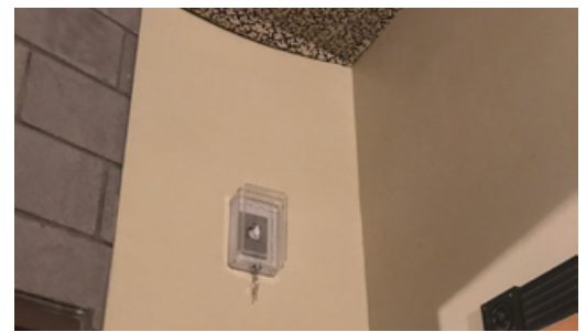
THE TIMER FOR THE LAMPS IS LOCKED INSIDE AN ACRYLIC CASE IN A SEPARATE ROOM, MOUNTED HIGH UP SO A STEP STOOL IS REQUIRED
