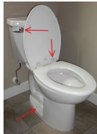
No build-up on hinges, flusher or base of toilet.
