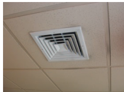
No dust/cob webs are visible on ceiling vents, corners, partitions and lights.
