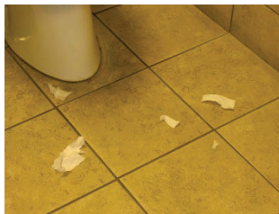
Debris on Floor
