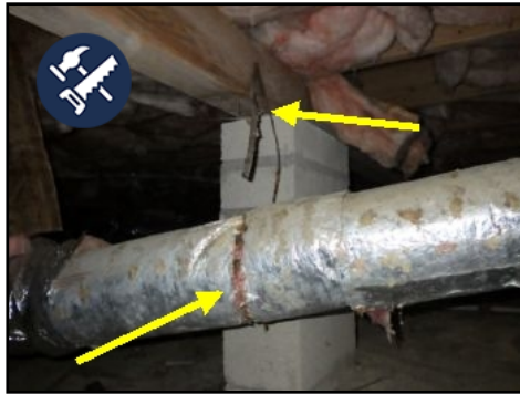
Fallen ductwork
