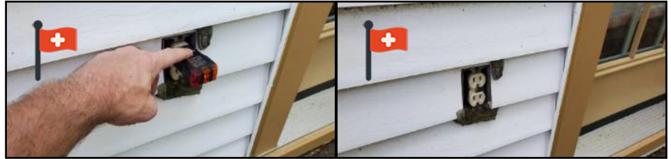
Add Exterior GFCI Outlet
