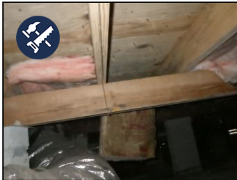
Fallen/missing Insulation
