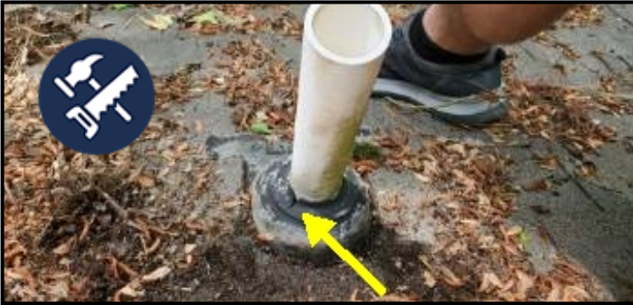
Cracked pipe boots
