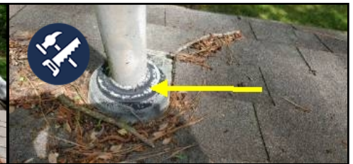
Cracked pipe boots
