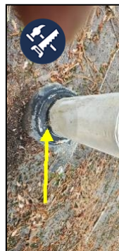
Cracked pipe boots
