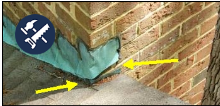
Damaged Flashing
