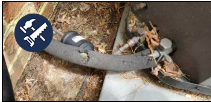
Damaged Insulation
