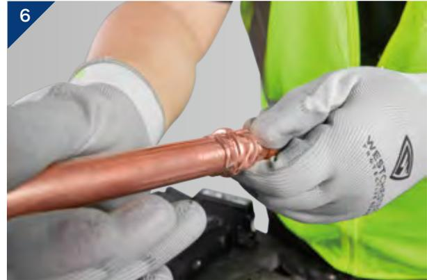
5. Press the fitting: Right jaw sizes should be used. Choose the correct jaw size, depress and hold the trigger of tool until the press cycle of the tool is fully completed. In addition, please refer to tool manufacturer’s operation manual for details of instructions.
