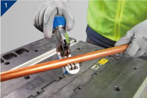
1. Cut the Tube: Tube should be cut completely square and there should be no defects and scratches on the tube which may affect the integrity of joints.
