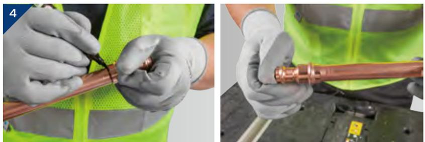
**MAKE SURE Fully Insert Tube and Mark Tube Insertion Depth**
