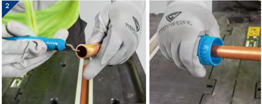
**MAKE SURE Deburr the Tube Thoroughly Inside and Out**
