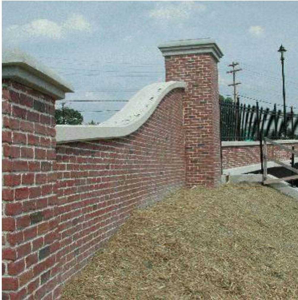
Figure 6. Formlined Concrete (photo courtesy of Custom Rock Formliner)
