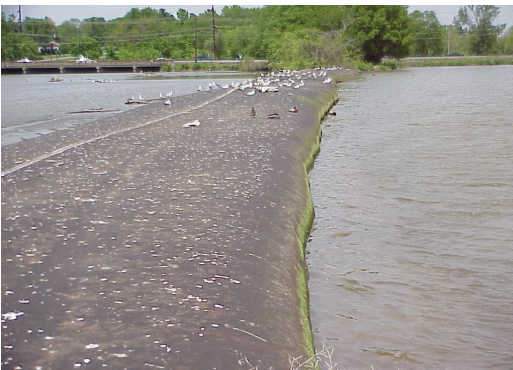
Left: Newly filled geotube. Initial public reaction was negative although the birds seemed to enjoy them. Right: 50' test planting area consisting of native wildflowers and grasses. Muskrat heavily grazed the area on the right side of the photo. Although this decimated the wildflowers, it provided an opportunity for the native grasses to emerge.
