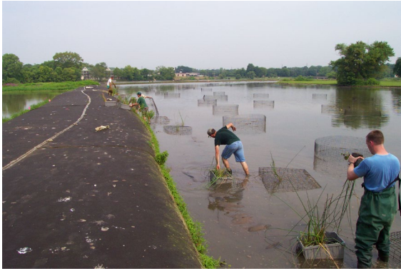
Left: TWRA, USDA, and Tennessee Tech volunteers assisting in planting aquatic vegetation in the upper end of the embayment. Two or three species were planted in each cage. Geotube is on the left. Right: Looking across the embayment at the geotube after one growing season.
