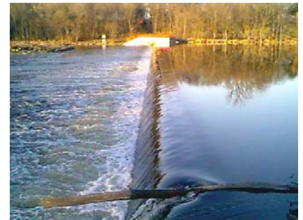
Yorkville Dam on the Fox River
