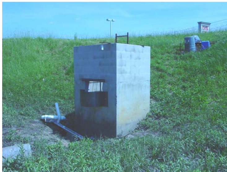
Figure 3. Modified concrete riser outlet.
