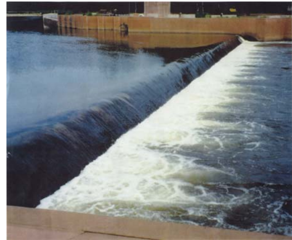
Example of a dangerous low-head dam built for water supply.
