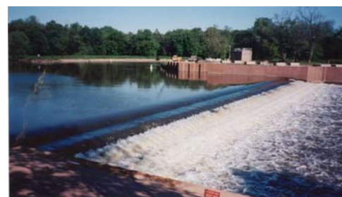
Killer dam tamed with stepped spillway.
