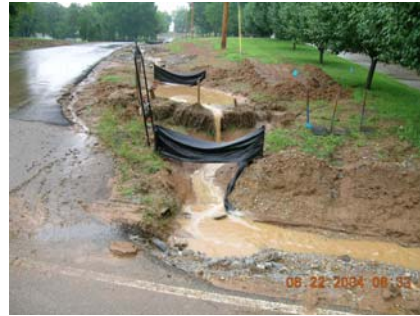
How not to install silt fence!
