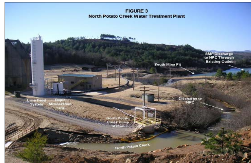
Figure 3. NPC Water Treatment Plant
