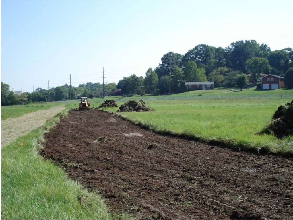
Figure 8. Stripping the grass from the area that will become the stormwater wetland. Note the mowed area on the left side of the photograph. That is the location of a sanitary sewer easement.
