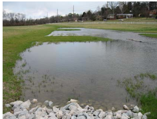
Figures 9 and 10. After views of the stormwater wetland taken three weeks and three months following construction. Note how well the wetland blends into the natural landscape in the photograph on the left. Water levels are high in the photograph on the right following a recent rain event.
