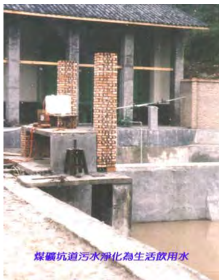
Figure 17. 300cum/d On Treating Wastewater from Coal Mine into Drinking Water. (China)
