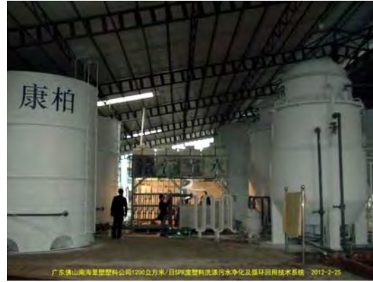
Figure 20. SPR System for 1200cum/day on plastics recycling industry. (2012.2 & 2012.3 CHINA)
