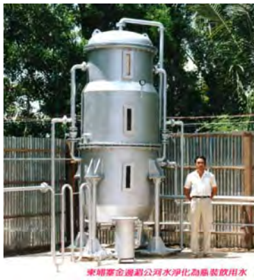
Figure 16. The SPR changes water of Mekong river into drinking water at Cambodia.
