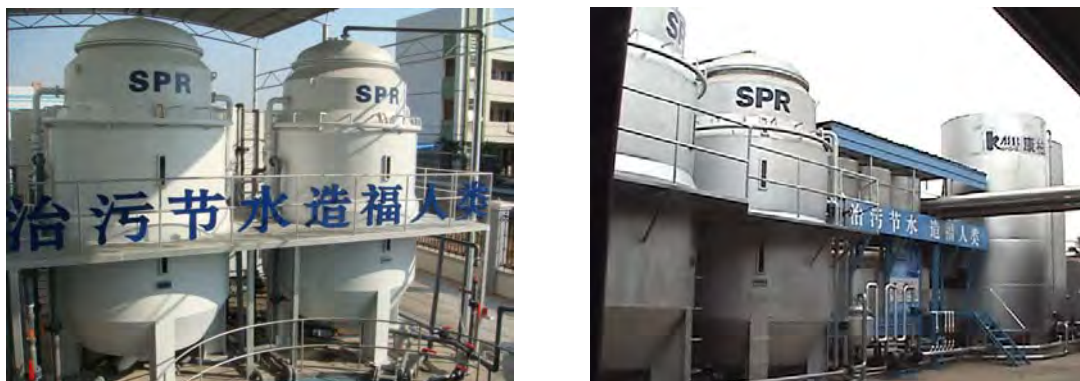
Figure 19. SPR System for 1200cum/day on textile industry (2005 & 2008 CHINA)
