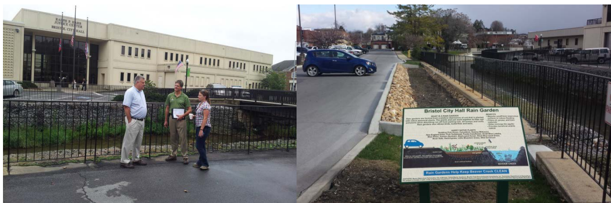
Figure 5. Before (left) and after (right) installation of raingarden. Parking lot runoff is intercepted and pollutants are trapped. Educational signage explains the process.
