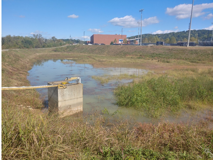
Figure 2. Detention basin following rainfall event.
