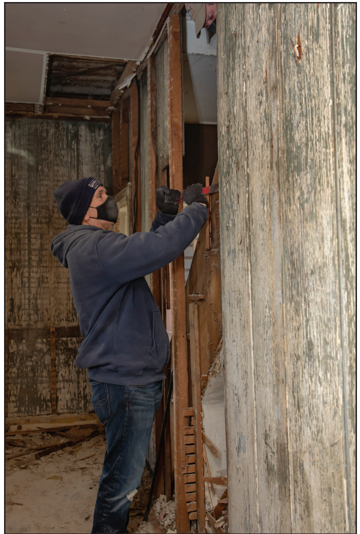
Bob Wheatley carefully removes original paneling. Courtesy of Paula Shannon.
