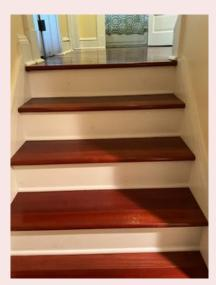
(I-3) Monitor: Left corner of first to second floor stairs appears to have old water damage. Using a moisture meter, did not see any current wet spots.
