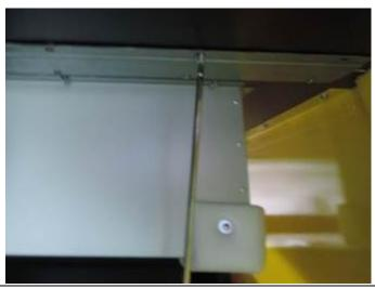
3. Fit a screw, spring washer, & flat washer to mount the metal bracket of Right and Left Metal Net
