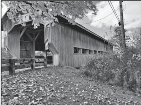
PHOTO BY NICK GROH/GOOGLE LOCAL The Caine Road covered bridge is the first Pratt truss bridge to be constructed in the state of Ohio.
