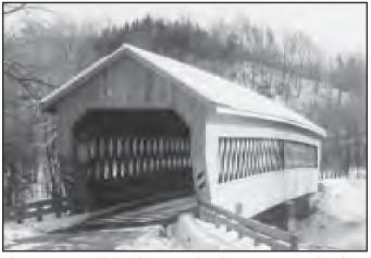
The State Road bridge was built in 1983 as the first "new" covered bridge constructed in the county. It has a Town Lattice design and clearance of 16 feet, 2 inches.
