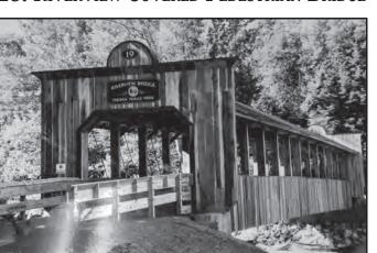
A wooden Pratt truss covered bridge built beneath the Smolen-Gulf Bridge, completed in 2016. The pedestrian covered bridge is 150 feet long and 14 feet wide. It is a Pratt truss design, like the Smolen-Gulf Bridge, and was designed by Smolen Engineering. It sits below Smolen Bridge in Indian Trails Park. It was dedicated on Oct. 4, 2016.
