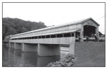
The Harpersfield Bridge built in 1868 is 228 feet long. It has a clearance of 12 feet and is built with Howe Truss construction. It is listed on the National Register of Historic Places. Renovated in 2022-2024.
