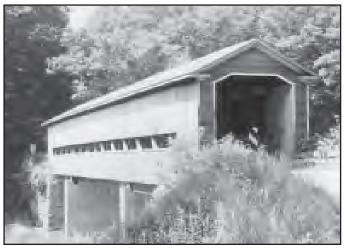
Middle Road Bridge was constructed in 1868 and reconstructed in 1984. It is 136 feet long and has a clearance of 11 feet. The bridge is east of State Route 7 and south of South Ridge Road.
