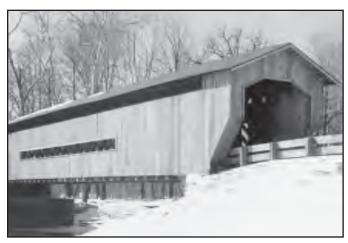
The Benetka Road bridge was built in the early 1900s. It is 138 feet long and has a clearance of 11-feet, 6-inches. The laminated arch was added during the renovation of 1985. It is on Benetka Road, which is off ŠR 193 north of Gageville-Monroe Rd.
