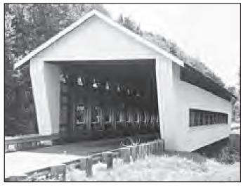
The Giddings Road bridge was built in 1995, east of SR 46 south of Griggs Rd. It is 107 feet long and has a clearance of 15 feet, 6 inches. It was built with Pratt Truss construction.
