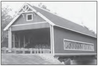
The Netcher Road Covered Bridge features neo-Victorian design with a timber arch and inverted Haupt walls. It was built in 1999. It is 110 feet long, 22 feet wide and features a clearance of 14 feet, 6 inches. It is east of Jefferson off Route 307 off S. Denmark Rd.
