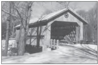
Doyle Road Bridge was built in 1868 on Doyle Road, east of Jefferson off SR 307. It has a clearance of 11 feet, 4 inches. It was rededicated in 1987 following the addition of a laminated arch. It is 94 feet long and features Town Lattice design.
