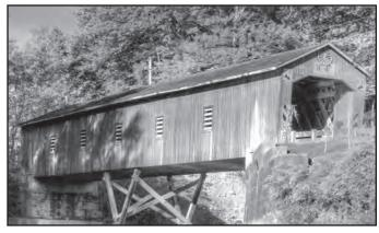
The Creek Road Covered Bridge was renovated in 1994. Its construction date is unknown. It sits 25 feet above Conneaut Creek and features Town Lattice design. It has a clearance of 9-feet, 3-inches. Creek Road runs east of Keefus Road, south off Route 20, in Conneaut.
