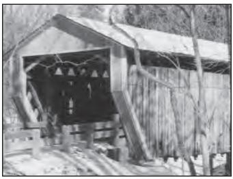
The Riverdale Bridge was built in 1874, with the floor rebuilt in 1983. The abutment was replaced in 1987. It has an 8-foot clearance. Riverdale Road is west of State Route 45, just past Camp Beaumont, in Morgan Township.
