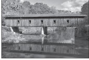
The Olin Covered Bridge is the only bridge named after a family. It was built in 1873 and features Town Lattice design. It is 115 feet long and has a clearance of 10 feet. It is on Dewey Road, east of Dibble Road, which is north of Plymouth Ridge Road.
