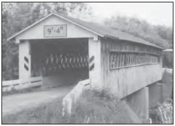
The Root Road bridge was built in 1868 and renovated in 1982-83. It is 114 feet long with a 10-foot, 6-inch clearance. It features Town Lattice design. Root Road is east of Stanhope-Kellogsville Road.
