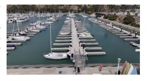
Bellingham is well into Phase 7 which includes half of west basin E-dock. The old dock has been removed and the new dock is already in place with piles driven. This is some quick work! Phase 7 is a little tricky and is being split out into two parts. The first part which they are working on now
