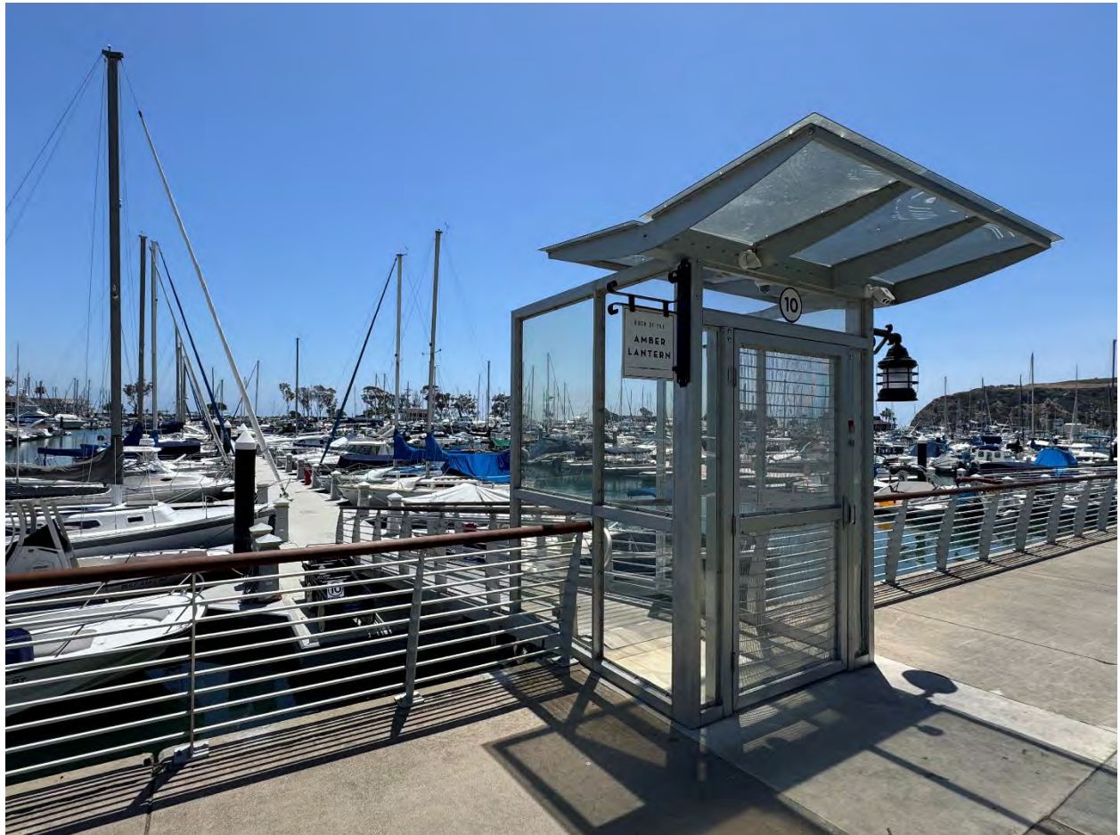
Image of New Gate, Railing, and Dock
