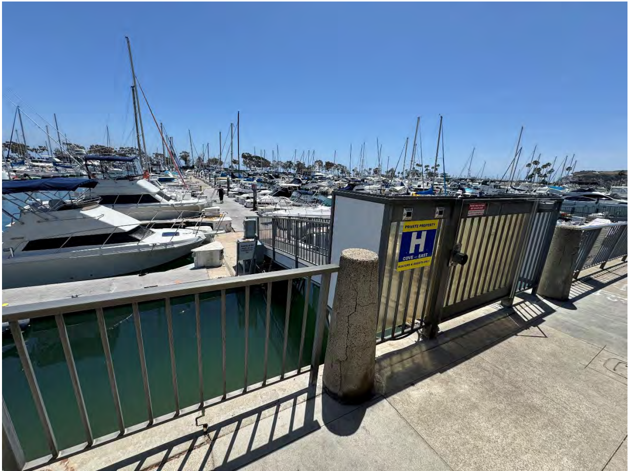
Image of Old/Existing Gate, Railing, and Dock
