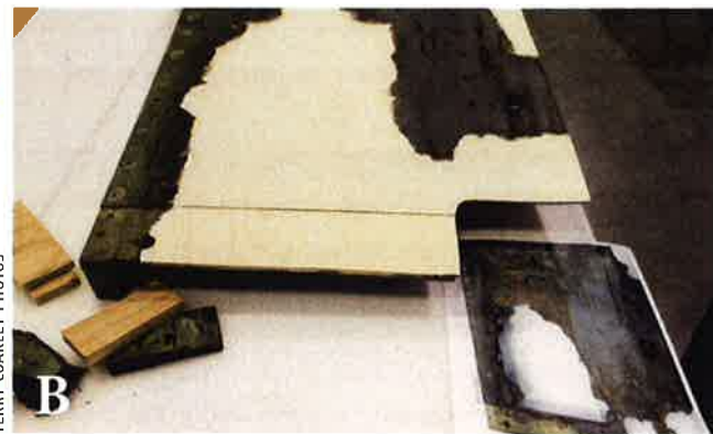
Three detailed views of the restoration project using plywood to fill in the gaps left behind by deterioration.
