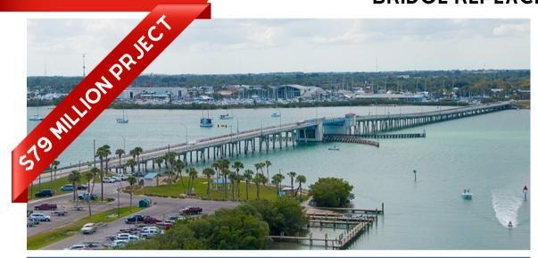
The existing two-lane 2,100-foot (ft) long Bridge, constructed in 1963 and includes a double bascule over the Intracoastal Waterway (ICWW) main waterway channel, is to be replaced due to structural deficiencies. The existing bridge includes two 10-ft 10-inch lanes, two 4-ft shoulders, and a 5-ft raised sidewalk on the north side. There are no dedicated bicycle lanes or barriers between vehicles and pedestrians.
