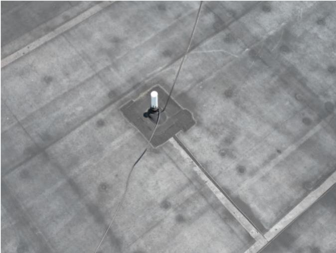
Sealant looks fairly new. Should be monitored/inspected annually for dry rot/cracks to prevent moisture intrusion.
