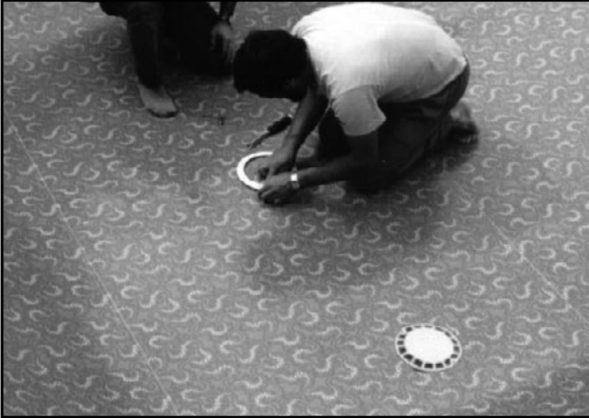
Optional main drain covers installation.
