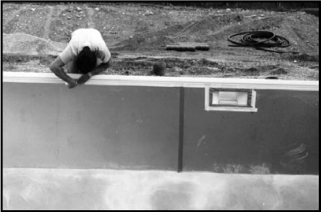
Tape off vertical wall seams.
