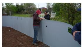
□ 3.6: As you unroll the wall, install **top rail (wall channels)** around the pool to give it more rigidity during installation. Ensure that the **top rail (wall channels)** are aligned with the **bottom wall channels**. To ensure a better stability of the wall during installation, use ropes, hooks and steel rods.
