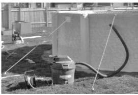
□ 5.2.5: To help the liner to fit the pool and remove the wrinkles, place your self along the wall, and with both feet do a slight jump a few inches backward while the vacuum cleaner is in operation. Do this all around the pool where there are wrinkles.
