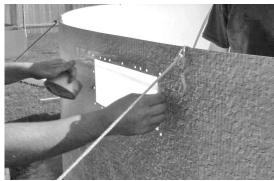
□ 5.2.4: Insert the hose of a vacuum cleaner a few feet into the water return. This will have the effect of pumping out the air and ease the process of removing the creases and wrinkles.
