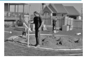
\* NOTE: If you install a geotextile (felt) liner protection for the bottom, you need to apply sand or crushed stone underneath the geotextile (felt). Do not put crushed stone directly under the liner.
