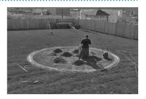
\* NOTE: A layer of 2 inches of sand is necessary to protect the liner from small rocks and pebbles. Consider enough sand to build the cove as well.
