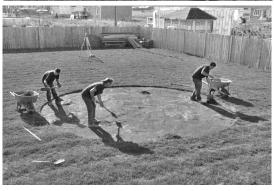
□ 1.2.4-B: IMPORTANT - FROST: In area where the ground freeze or the drainage is deficient, we recommend to add 2 inches of crushed stone by 18 inches width. This band of crushed stone has to be leveled and compacted and has to lie underneath the pool wall.
