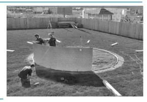
□ 3.5: Guide the wall in the **bottom rail (wall channels)**until both ends meet.
