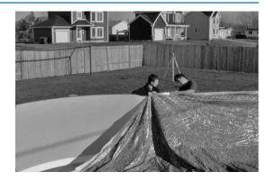
\* NOTE: Do not install the liner on both sides simultaneously. Be careful not to create wrinkles. Install the liner from one point to the end by following one direction.
