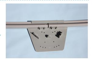
□ 2.4: Verify the height of each **bottom connector plate** with an optical level. They have to be at the same height. Adjust height if necessary.
