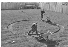
□ 1.2.4: Level the site using a shovel, a rake and an optical level. Remove all high spots and level to the lowest point within the boundaries. DO NOT ADD ANY SOIL TO THE SITE! Added soil will not provide the strength required to support the weight of the pool. The ground must always be firm. The entire bottom must be smooth and free of stones, sticks and any other foreign materials that could puncture the liner.
