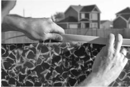
□ 5.2.2 - B2: Overlap the liner at the top of the wall and hold it in place by inserting the plastic coping.
