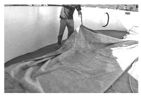
□ 5.1.1 – B2: Cut the felt along the base of the wall.
