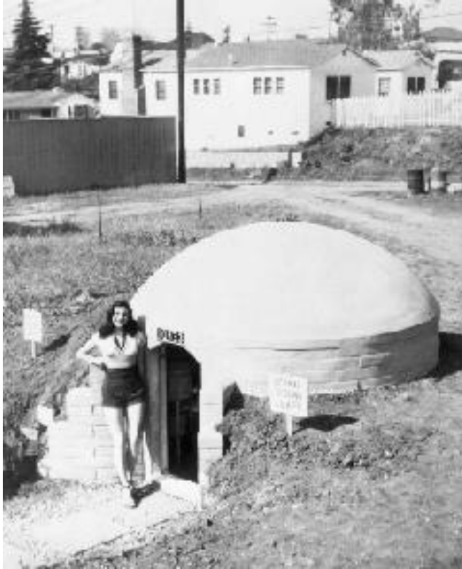
A backyard fallout shelter in San Francisco. (Bettmann/Getty Images)
