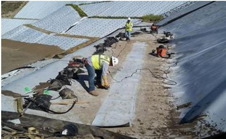
Installing Bowerman's landfill liner
