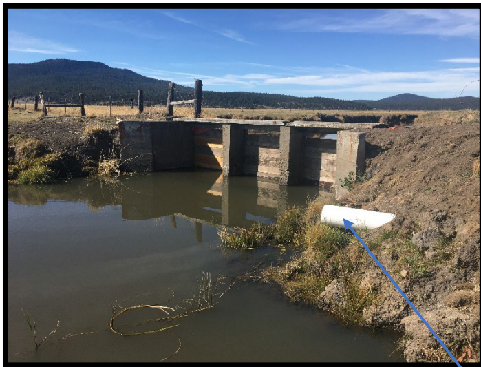
Exhibit 1: October 2019 – Irrigation Diversion looking upstream to the northwest. Boards are in place to divert water to meadow. White tube is a fish return pipe connected to fish screen.
