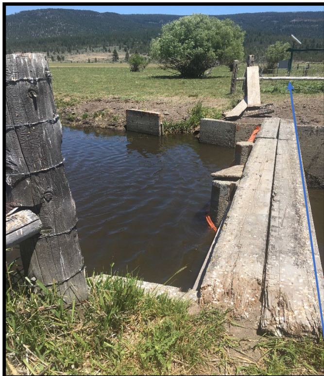
Exhibit 4: June 2020 – Photo showing irrigation water intake and fish screen.
