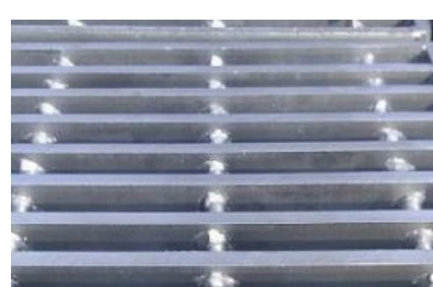
Swage-Locked Grating
