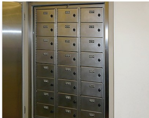
EXAMPLE 10B: Pass-through Temporary Refrigerator (Open front view)
