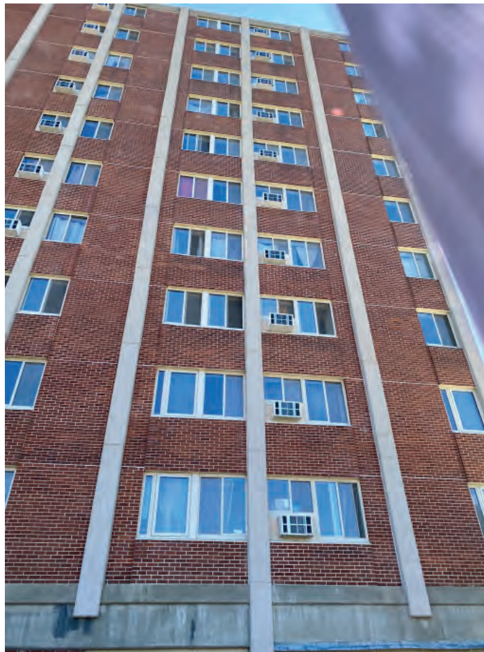
8. 11-story north wall brick repair completed between Columns 11-6 and 11-1.
