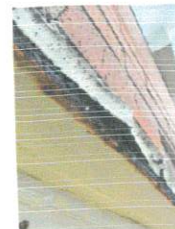
Lintel corrosion
