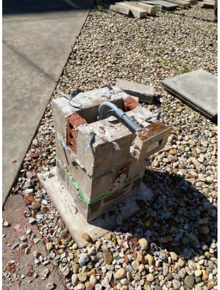
16. Some CMU block removed at piers.
