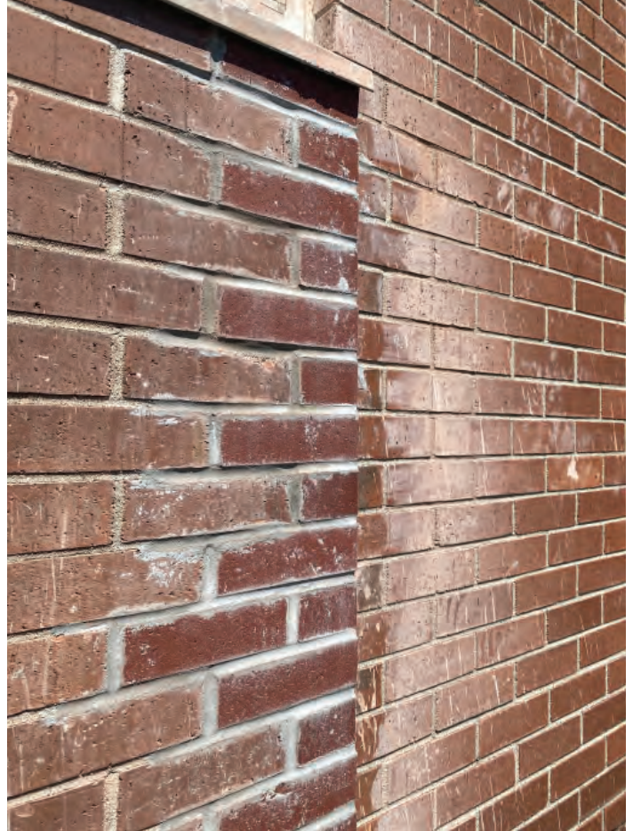
2. 11-story south wall brick replacement at window bump-outs (typical).
