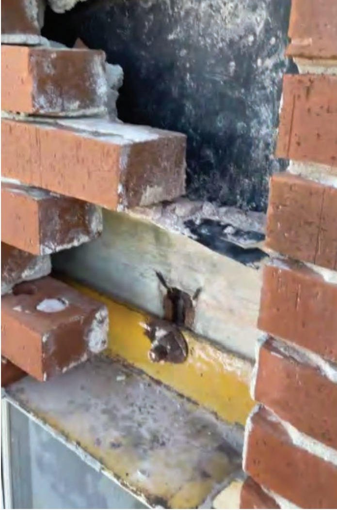
5. Opening at lintel.
