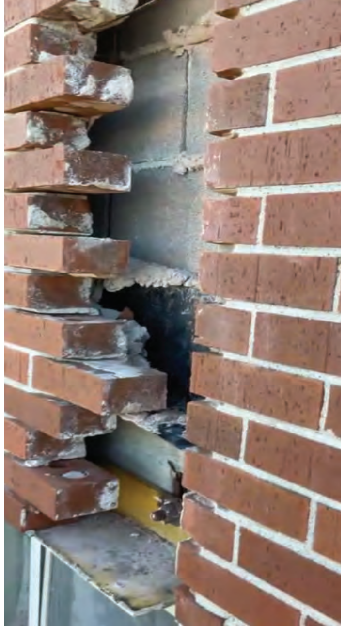
4. Opening above lintel.
