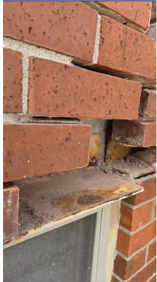
2. Lintels are not significantly rusty at the upper level.
