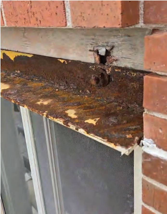
1. Lintel with acceptable thin layer of rust.
