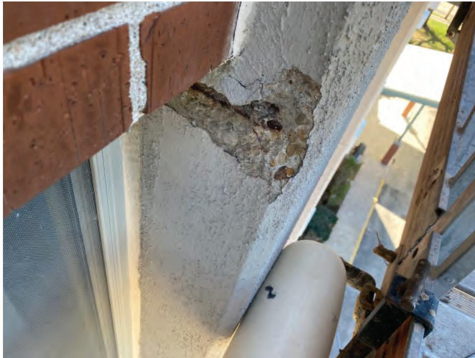
11. 11-story north wall significantly cracked concrete uncovered left of Column 11-8 above 5th floor window.
