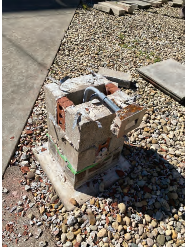
16. Some CMU block removed at piers.
