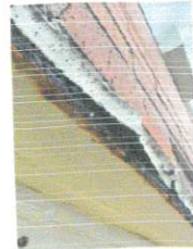
Lintel corrosion
