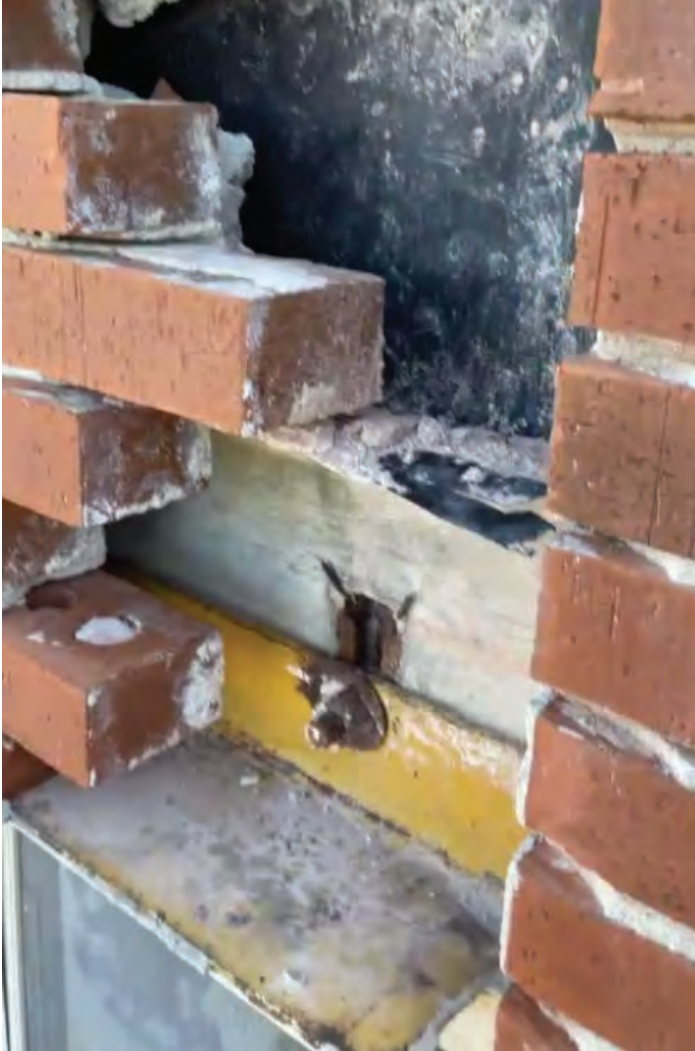
5. Opening at lintel.
