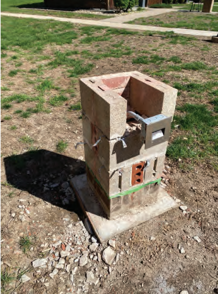
15. All brick removed from most of the piers.
