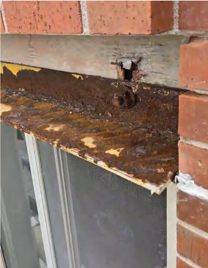
1. Lintel with acceptable thin layer of rust.
