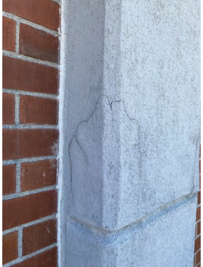
10. 11-story north wall area of additional concrete repair (typical).
