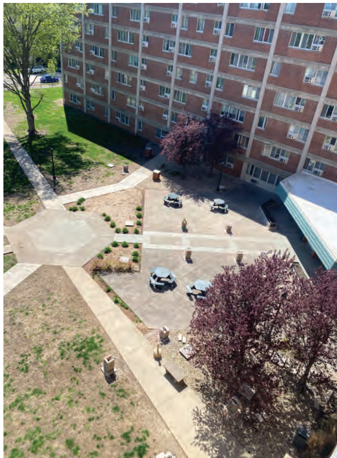
12. Progress of brick piers and planters.
