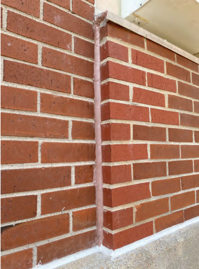
7. 8-story east elevation replaced bump-out brick.
