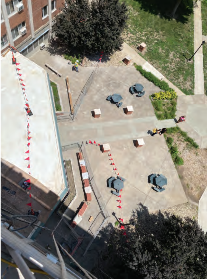
11. Brick repair complete at piers and in progress at planters.
