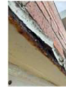
Lintel corrosion
