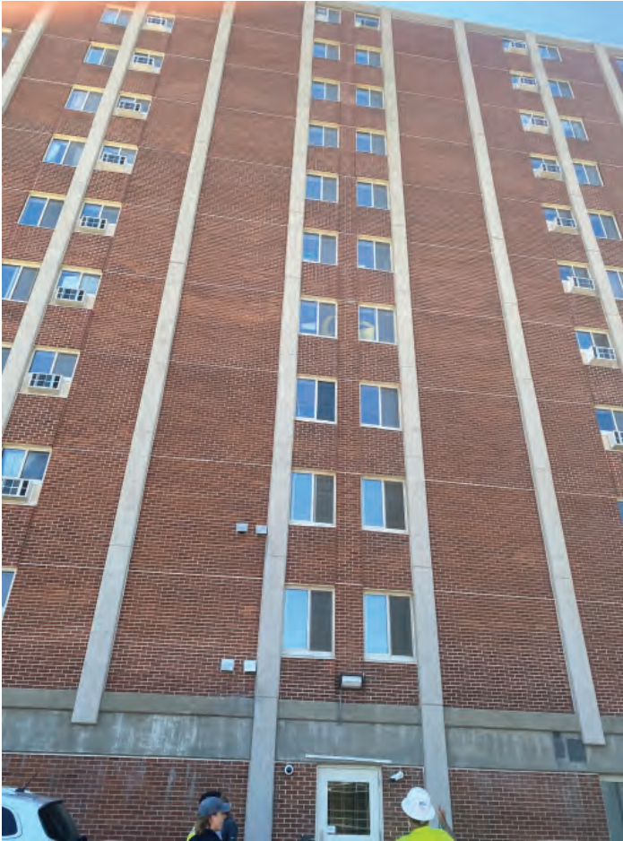
1. 11-story north elevation work complete.
