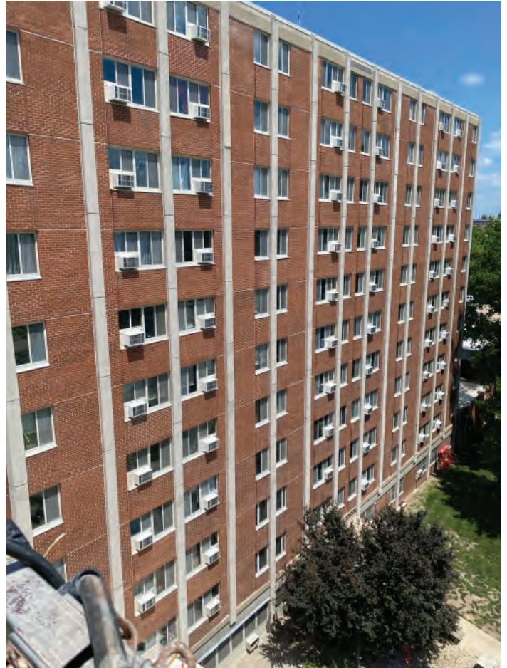
2. 11-story south elevation work complete.
