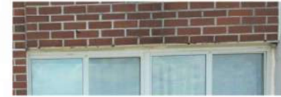
Lintel corrosion
