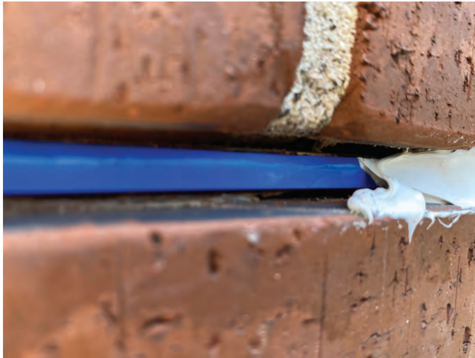
5. 8-story north elevation resealing shelf angles in progress.
