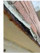
Lintel corrosion
