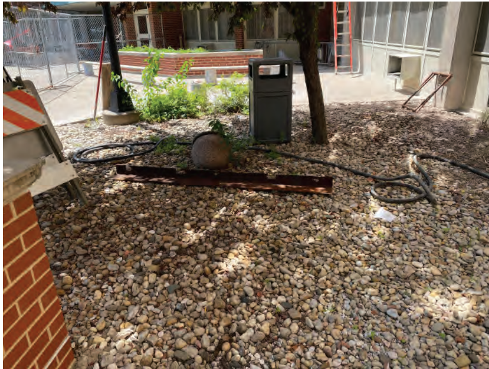
3. Single lintel that was replaced at the 11-story building.
