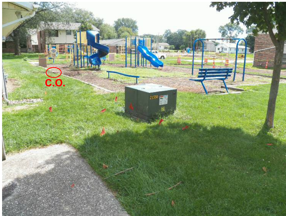
6. C.O. location at Community Building.
