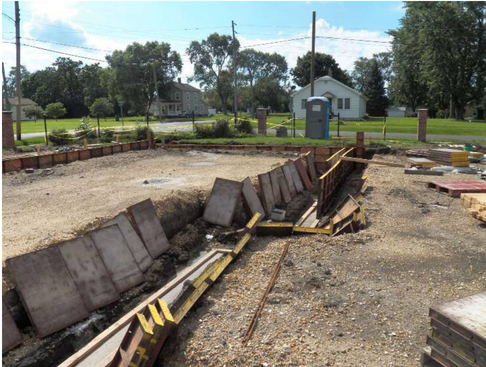
1. Building B-HC-2 looking southeast.
