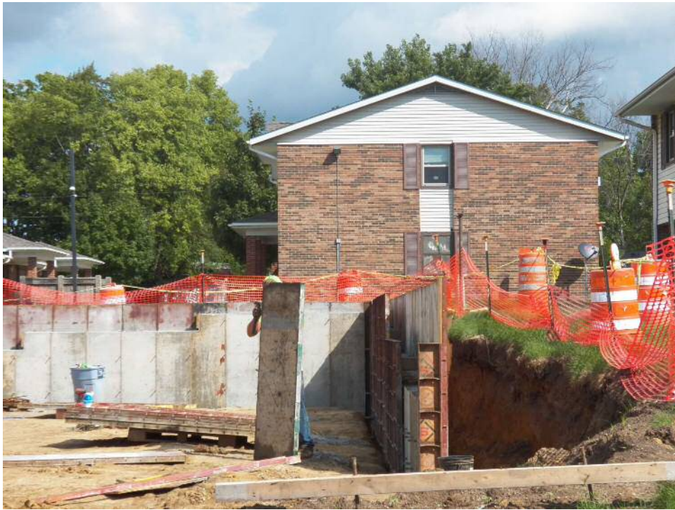
5. Retaining wall at basketball court.
