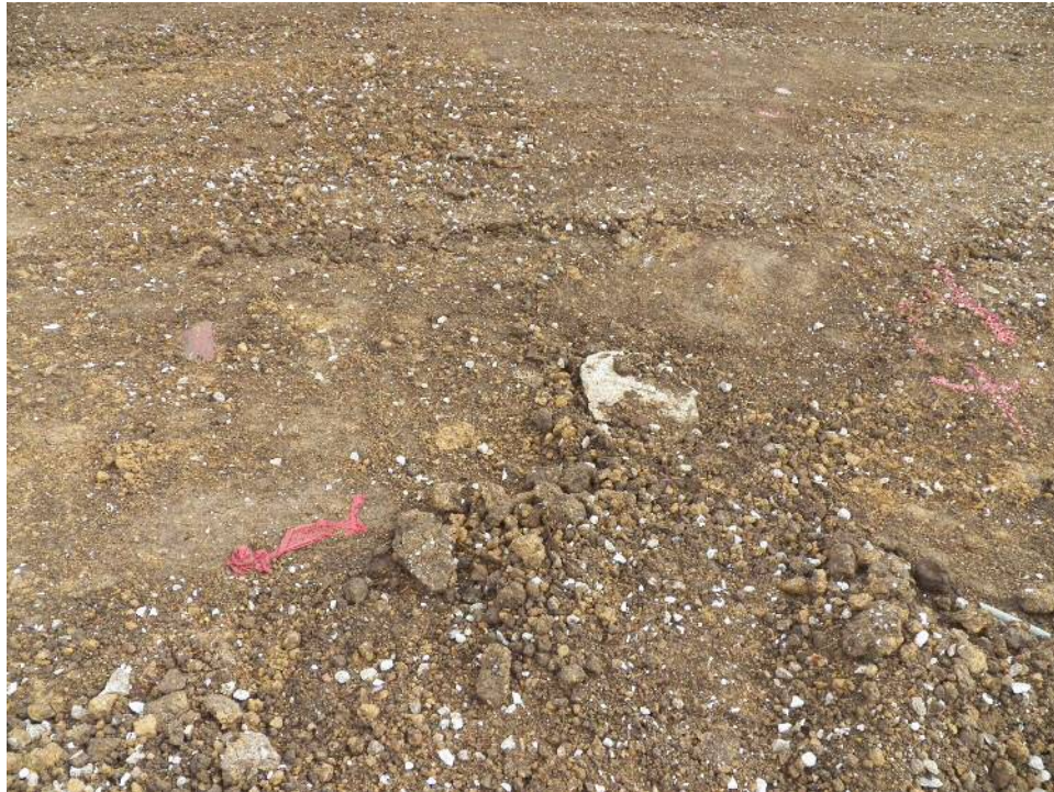
6. Organic soil at basketball court.
