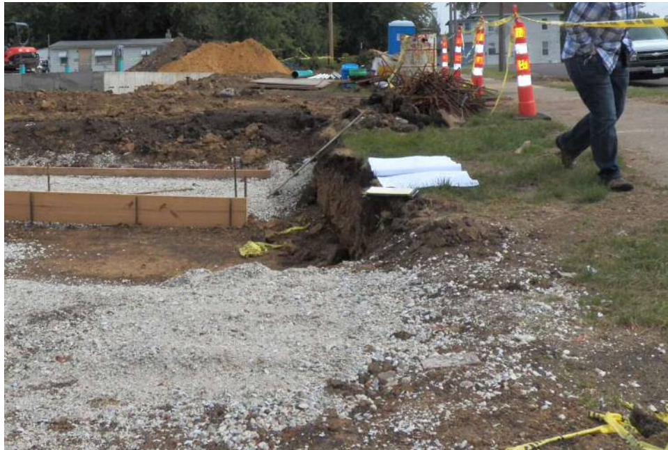
4. Grade at southeast corner of parking lot addition.
