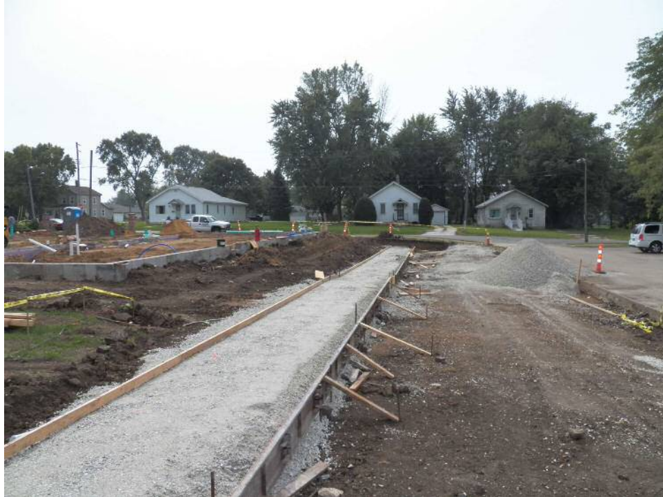
1. Parking and Building B-HC-1.
